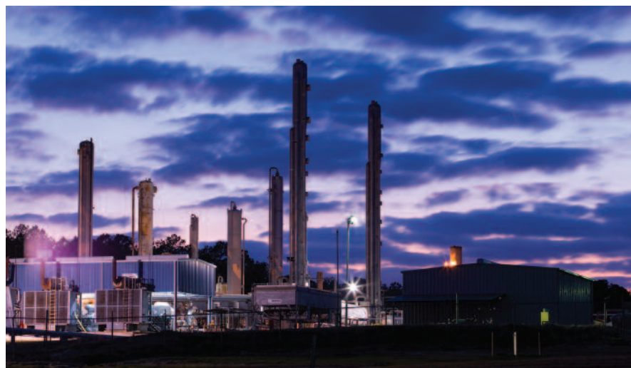
Eagle Rock owns 1,195 miles of pipeline, 43,700 horsepower compression and seven processing plants in the Haynesville Shale, Deep Bossier/Angelina River and Austin Chalk plays in East Texas, including both the East Texas main line that runs north and south and the Brookeland system that runs east and west.
